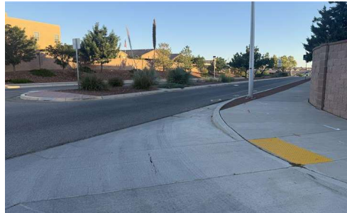
Figure 4: Sight Distance looking Right on Fairbanks Dr
