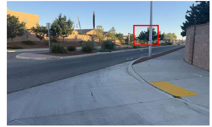
Figure 7: Sight Distance looking Right on Fairbanks Dr
